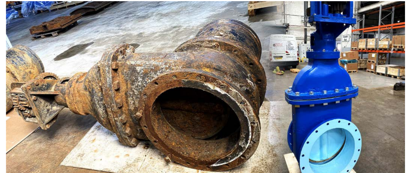
Munnoch Reservoir 24" Gate Valve Replacement Before And After
