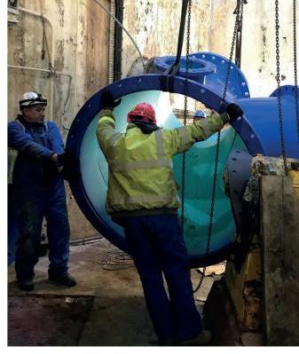
The logistics of the project were far from straightforward. The pumping station is 8m below ground, in line with the base of the dock. This is common practice with dry docks as it optimises pump efficiency. Once a ship is in place and the dry dock gates are closed the water is pumped out and returned to the Clyde at low tide.
