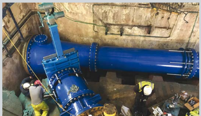
Installation of new pipework, electrically actuated knife gate valve, flange adaptor, and slanted seat check valve
