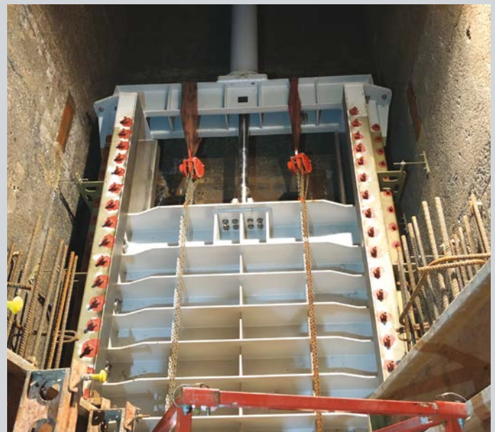
Secondary Scour Gate in position
