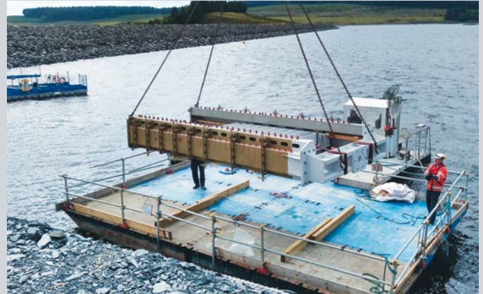
Bulkhead Gate being loaded onto Pontoon for transportation to Intake Tower
