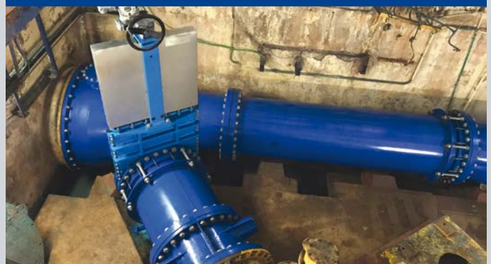
Installation of new pipework, electrically actuated knife gate valve, flange adaptor, and slanted seat check valve
