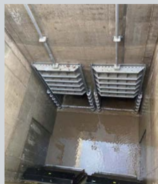
Installation of Wall Mounted penstocks
