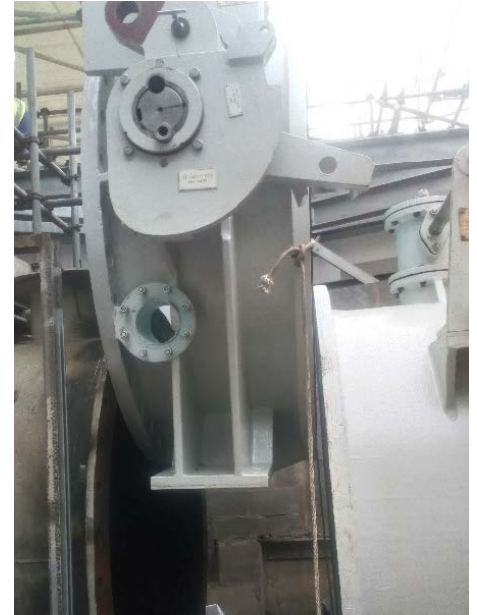
Installation of refurbished butterfly valve
