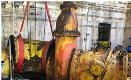
Extraction of the old pipework, gate valve and check valve
