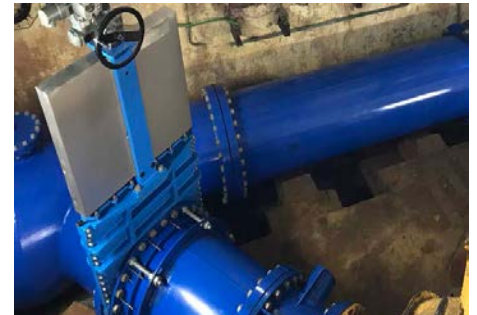
Installation of new pipework, electrically actuated knife gate valve, flange adaptor, and slanted seat check valve
