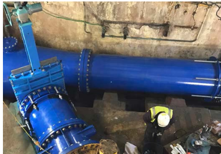
Installation of new pipework, electrically actuated knife gate valve, flange adaptor, and slanted seat check valve
