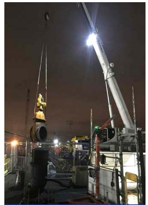
Existing Gate Valve being removed
