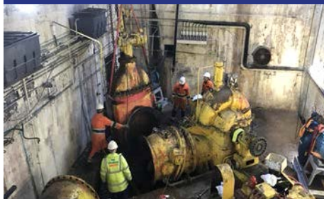
Extraction of the old pipework, gate valve and check valve
