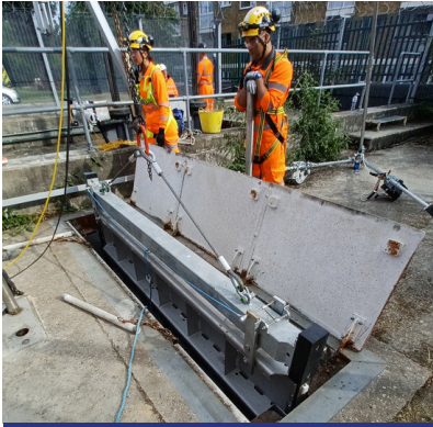
Lowering the new stainless-steel chases
