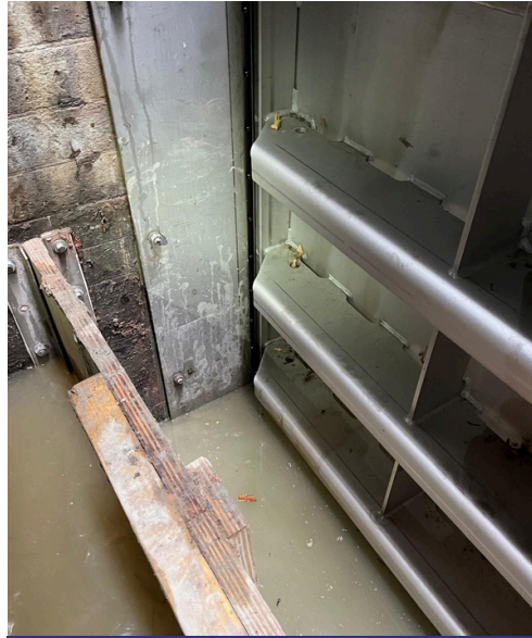
Stainless-steel chases in position
