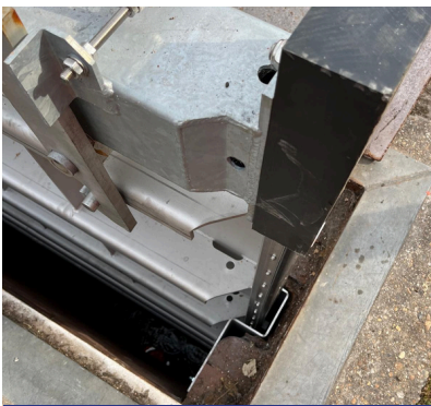
Lowering the new stainless-steel chases
