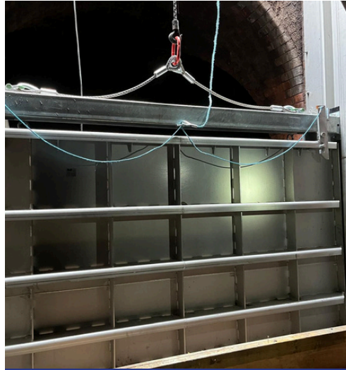
Lowering the new stainless-steel chases
